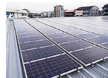
Solar panels installed on the roof of a Kanagawa Nissan dealership. Power from the panels is supplied to dealerships through the Nissan PPS system.
